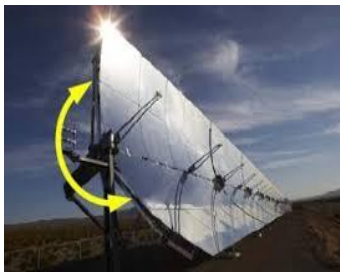
Figure 2: solar tracking system
